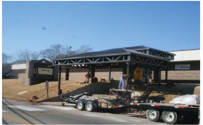
Pictured above is work progressing at the Lance Elementary Entry Area.
