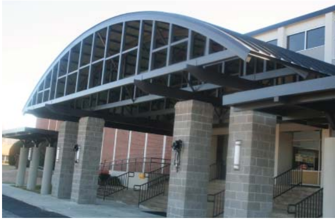
Pictured above is the new unloading area at Lanett High School
